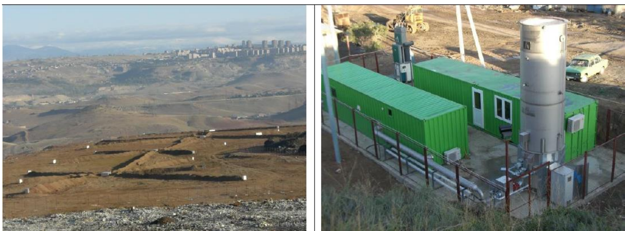
Figure 5.1. Distribution of methane extraction wells in Nubarashen landfill “Block B-Western” site (on the left), methane flare plant (FP, on the right)
